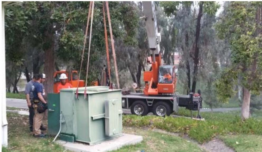
The current T-76 transformer near the Interim Classroom Facility broke down, and in an effort to help prevent future failure, the Facilities Management high voltage group and staff from the Central Plant replaced the transformer.
