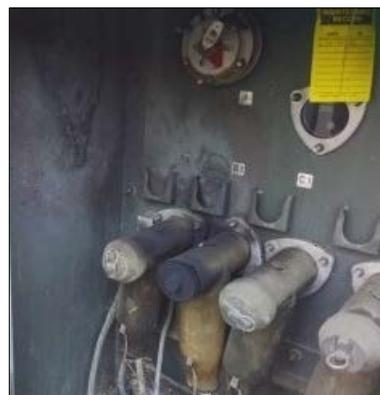
T-Body Failure in High Voltage SF-6-19A
