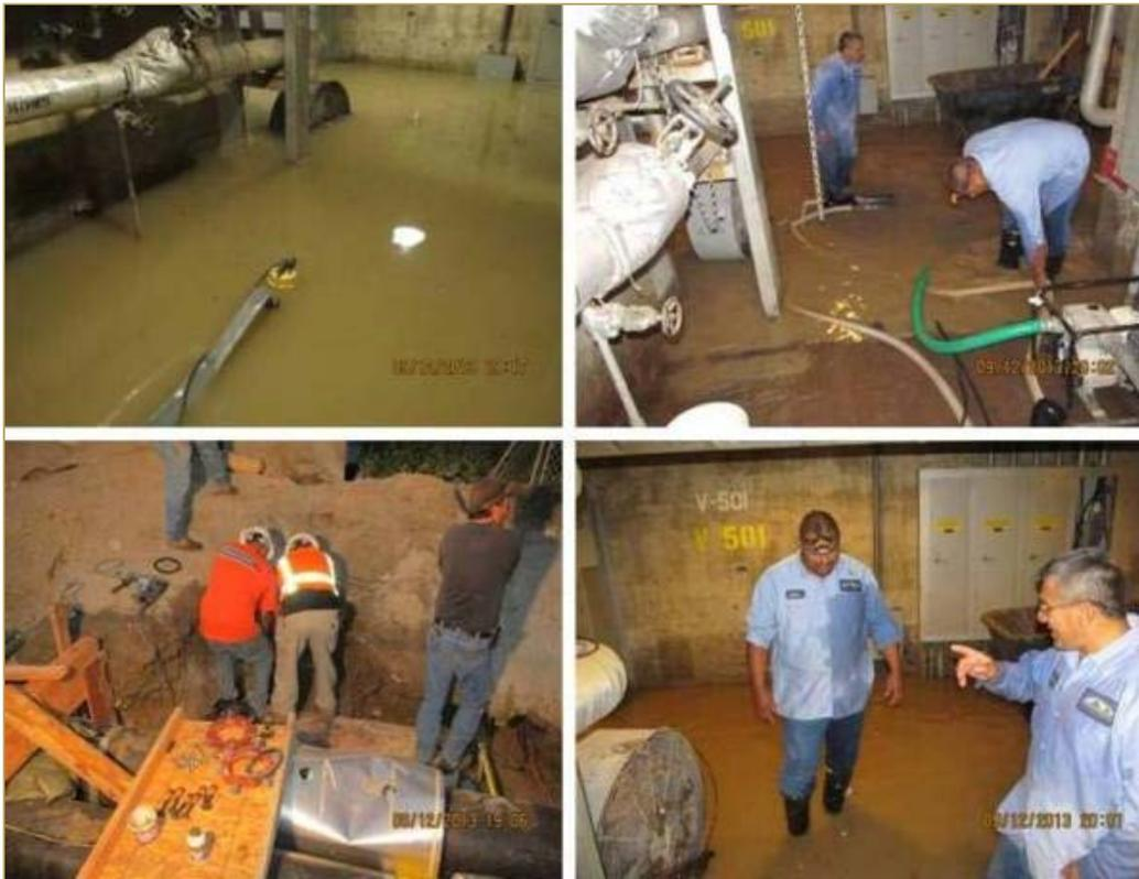
In September, Facilities Management responded to a water line rupture that began to flood the utility tunnel during the construction of Business Unit 2. This tunnel houses the campus high voltage (12,000 volts) distribution system and other crucial campus infrastructure.
